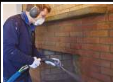
Wood and Brick Cleaning
