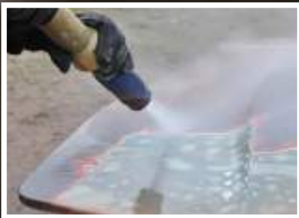
Coating and Paint Removal
