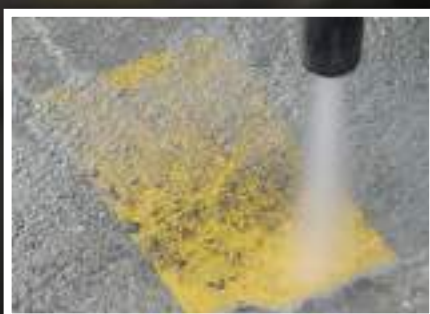
Concrete Cleaning and Surface Preparation
