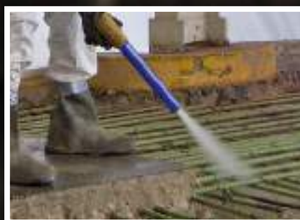
Concrete Repair and Restoration
